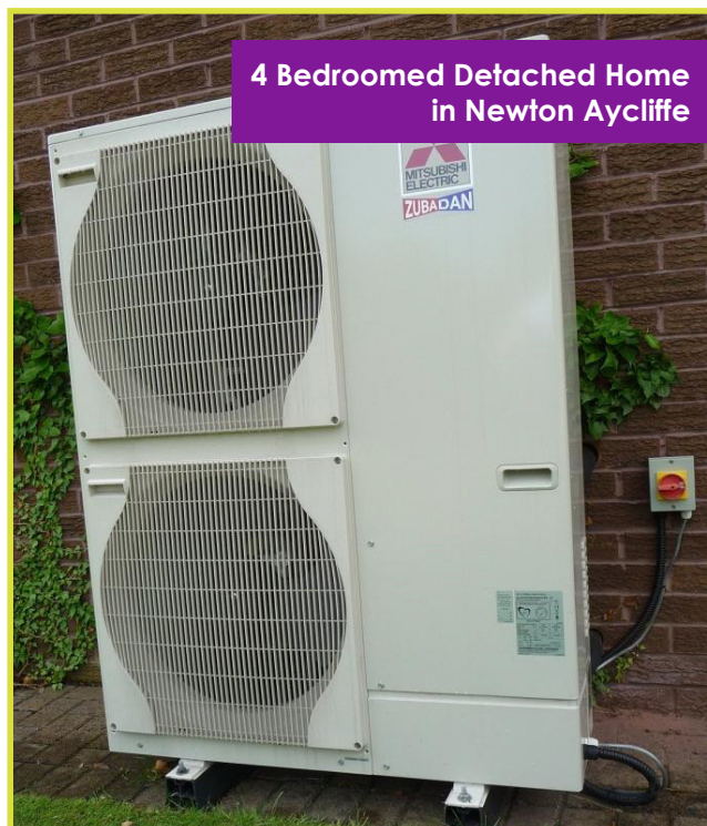
Above: Showing the Air Source Heat Pump outside the house
