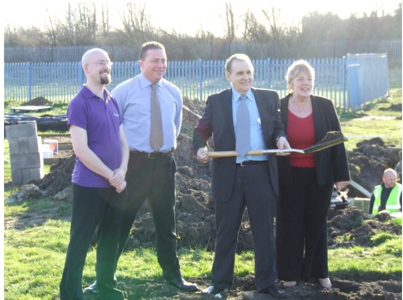
The above picture is of the official ground works opening ceremony on the 28 th January 2008. Pictured are from left Dr Matt Hogan (Revolution Power Director), Gavin Hill (Terra Nostra Manager), Cllr John Sterling and Carole Bell MBE (Meadow Well Centre Manager).
