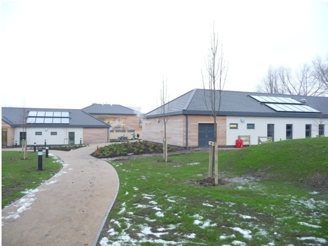
Above: Schuco Compact Line Solar Thermal Water Heating System installed with a 'in-roof' Kit. The kit is installed after the felt and latts are installed prior to the tiles.
